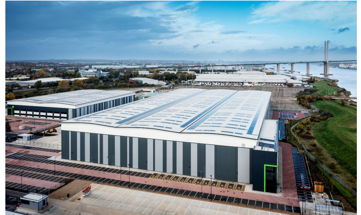
Crossways Commercial Park, United Kingdom
