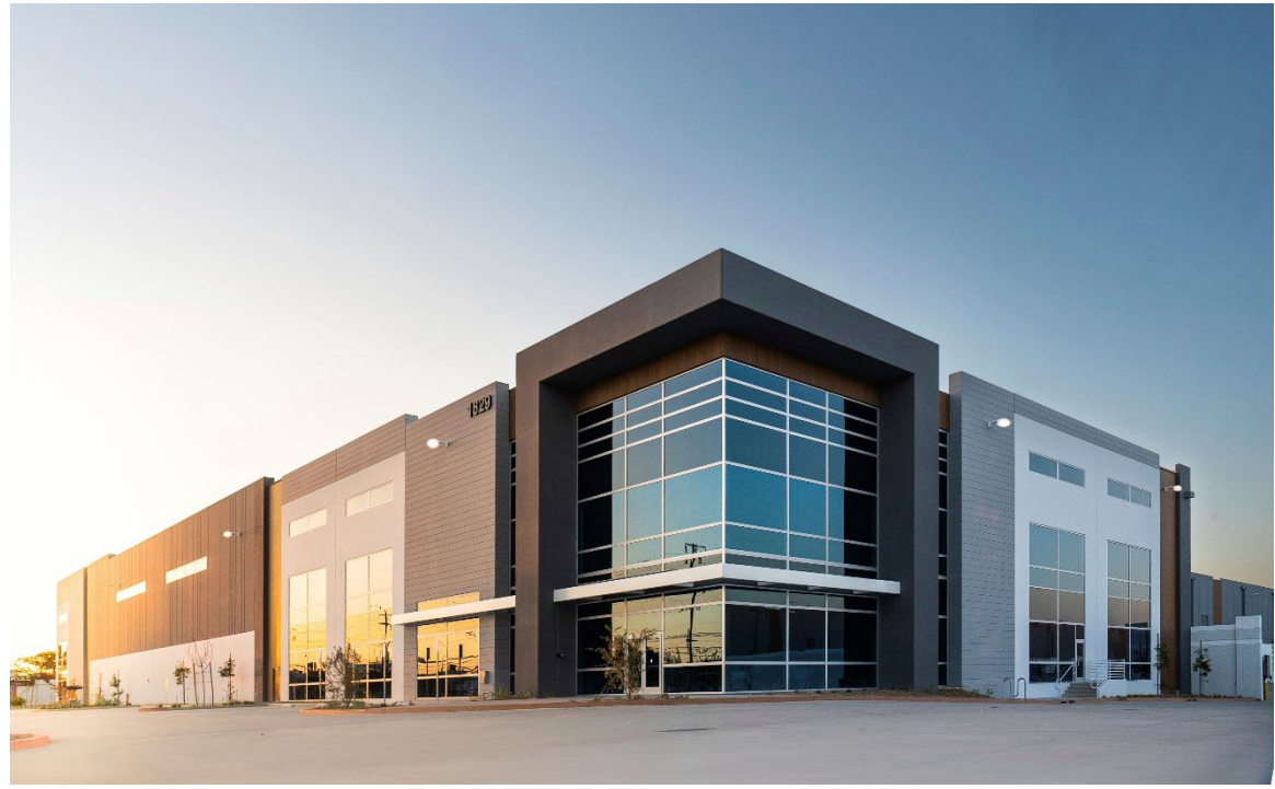
Goodman Logistics Center Fullerton, Los Angeles, USA.
